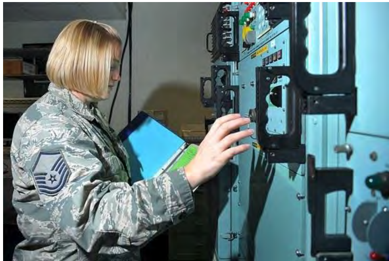
Strategic Automated Command Control System, Offutt AFB, NE
