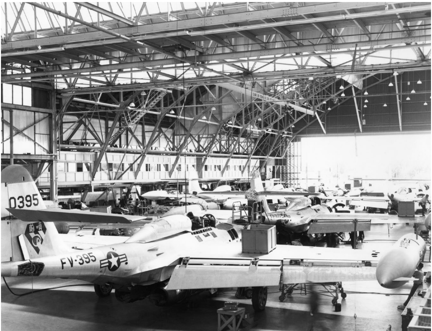
F-89 aircraft depot maintenance line, Hill Air Force Base, 1953.
