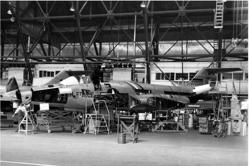
This June 1959 photograph shows an RF-101 jet reconnaissance aircraft repaired under the Time Compliance Technical Order (TCTO) system, which augmented the more comprehensive Inspect and Repair as Necessary (IRAN) depot maintenance process.
